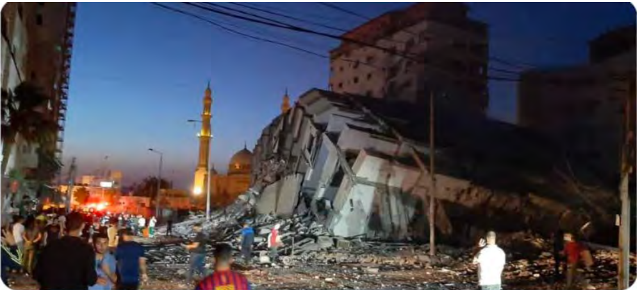
Two cases of damage inflicted by the IDF on the infrastructure used by Hamas leaders
